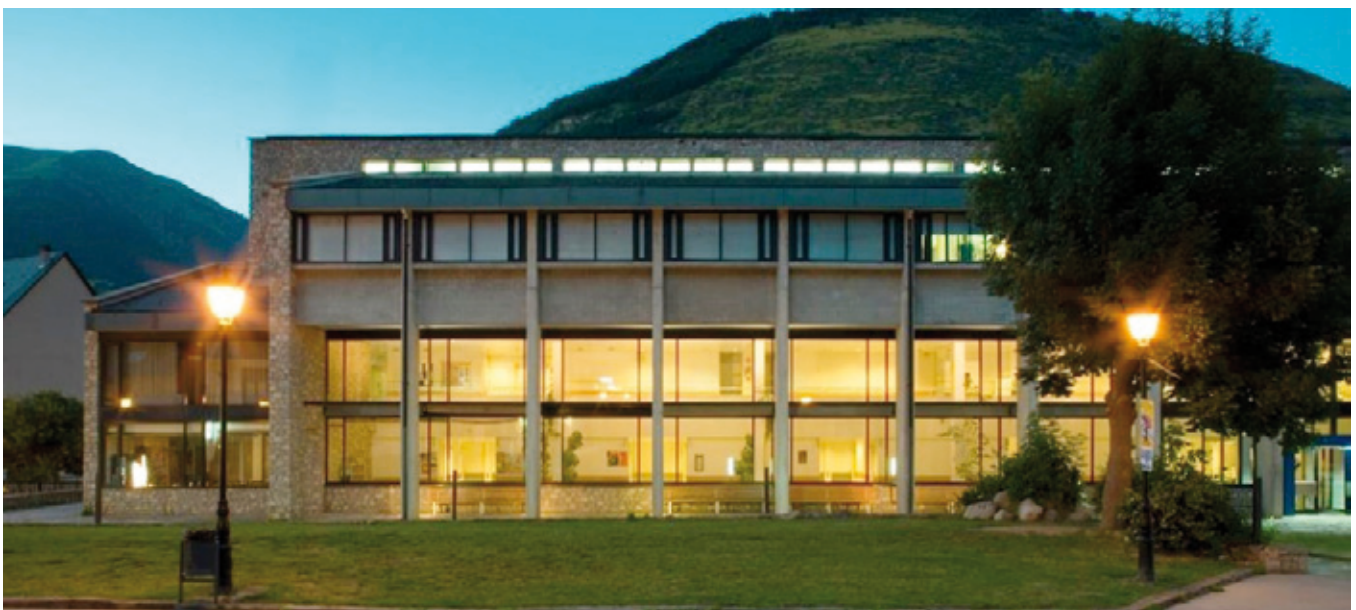
Access Control with IP System in Viella Hospital (Spain)
