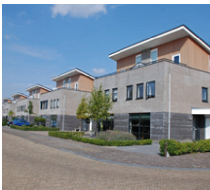
Multiple facilities control through a checkpoint
