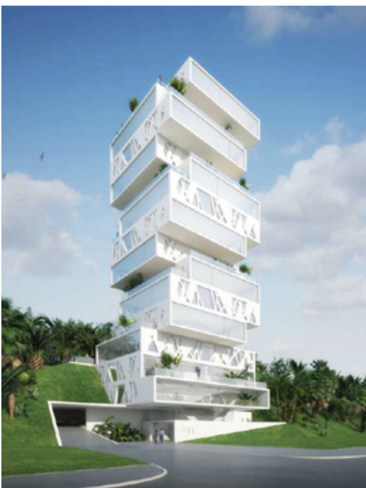
Tactile Monitors & Alea entry panel in The Cube building (Lebanon)
