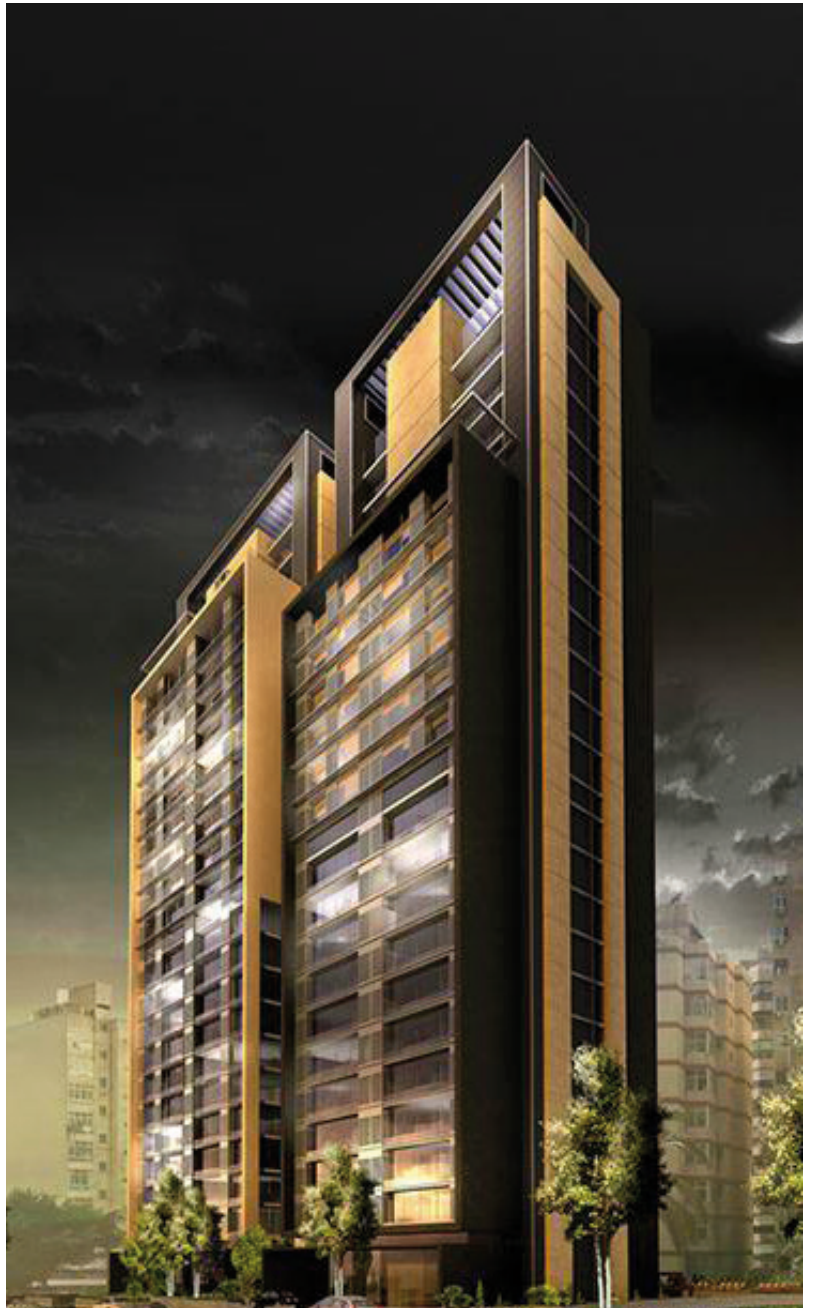
Tactile Monitors & Alea entry panel in Titanium Towers (Lebanon)
